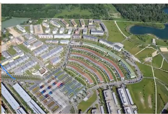
Solar City, by Atelier Dreiseitl, in Linz-Pichling, Austria
